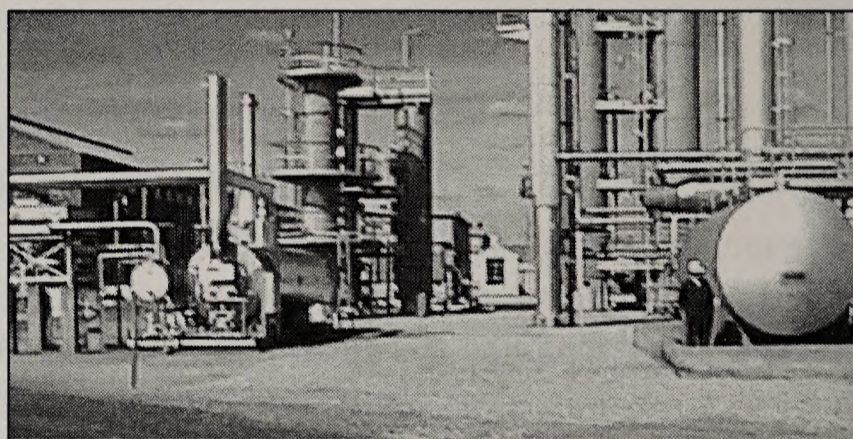
Figure 4: Work area between the reclaimer and the MEA tank, after cleanup.
